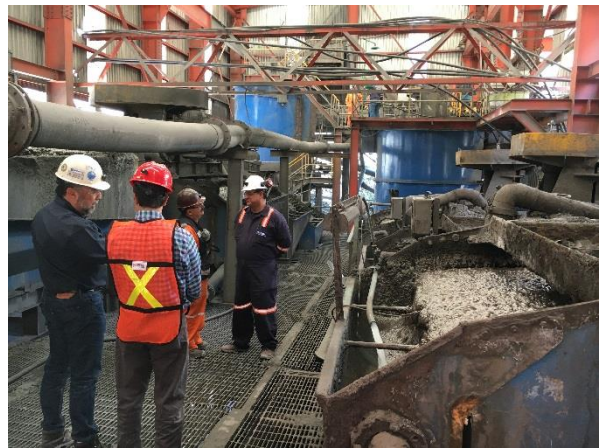
Photo 6 – Pb-Cu flotation and conditioner tanks.
