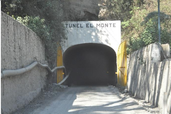
Photo 1 – El Monte Mine portal entrance, located at the Monte Beneficiation Plant.
